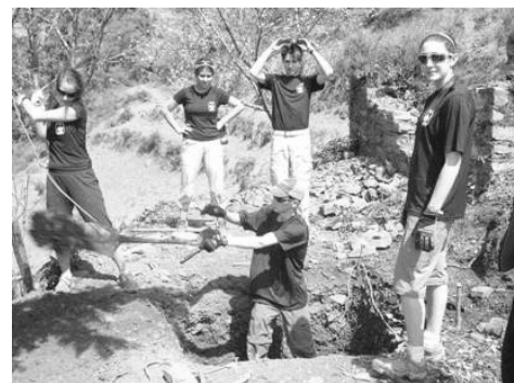
Nobles Students Dig a Soak Pit
